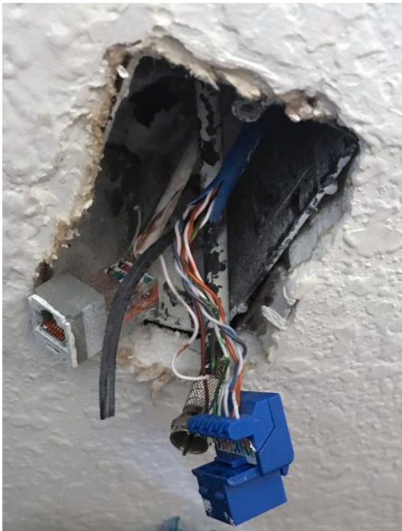
Figure 1: a student apartment wall jack after several years of painting and repairs
